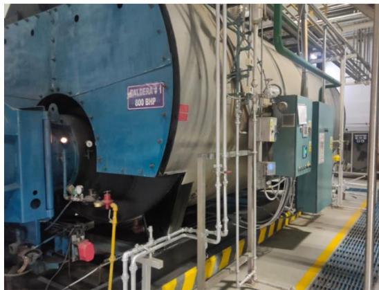
**Figura 2. 2:** Caldera pirotubular horizontal
