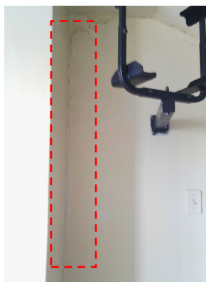
Figura 18: Fisura Vertical
