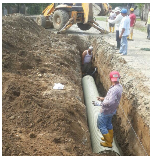
Figura 15: Colector secundario \varnothing 650mm
